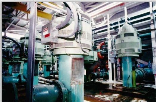
Motor powering matrix booster pump in a phosphate mine
