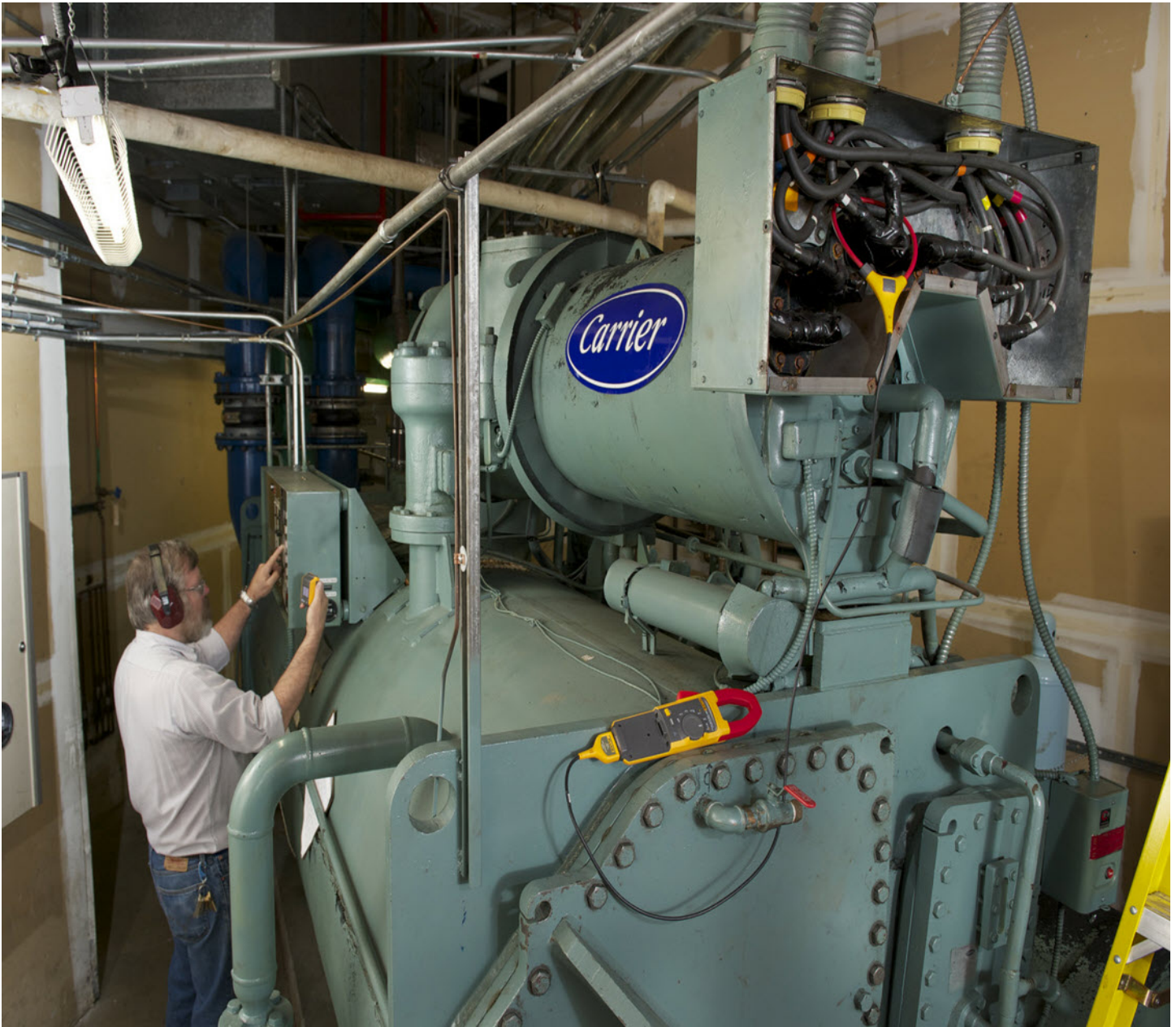
Fluke 381 with iFlex, remote display is in technician's hand
