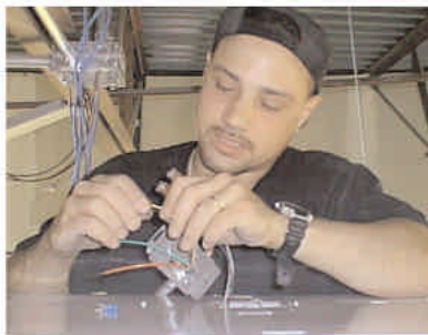
WAGO WALL-NUTS™ work with solid and stranded wire making main, branch and fixture hookup fast, easy and safe.
